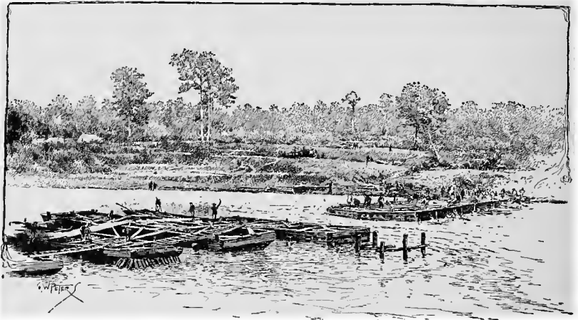
Building the Dam on Red River which released the Fleet.
